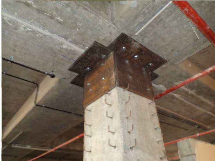
Figure 4 – Collar after installation (WIDIANTO, 2006) (8)
