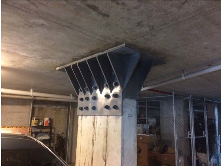
Figure 4 – Collar after installation (WIDIANTO, 2006) (8)
